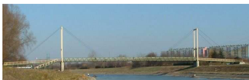
d) footbridge in Tropie main span 110 m
