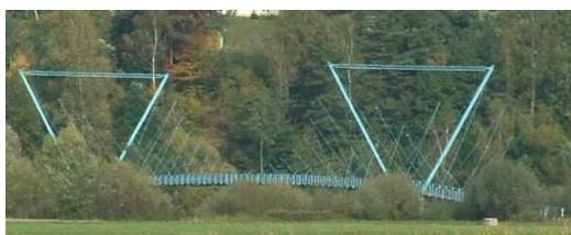
d) footbridge in Tropie main span 110 m
