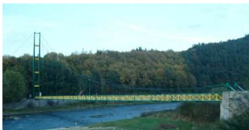
c) footbridge in Rzeszow main span 64 m
